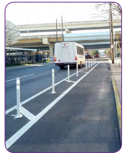
Figure 3-5 Class IV Buffered Bicycle Lanes
