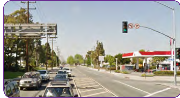
Figure 4-5 Looking north along Fairview Road at Newport Boulevard, no existing bicycle facilities
