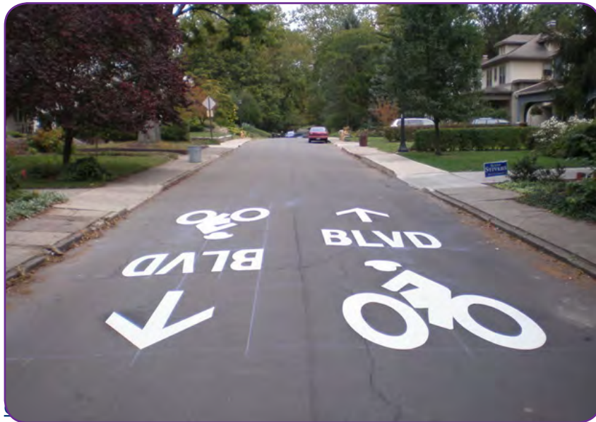
Figure 3-8 Class III Bike Boulevards
