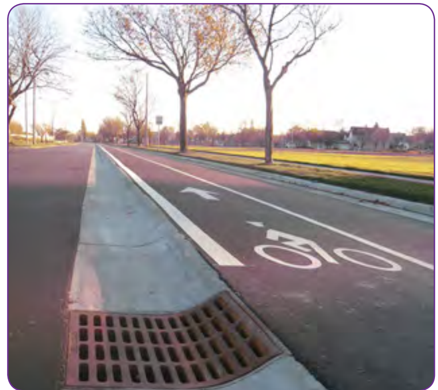
Figure 3-11 Class II Raised Bicycle Lanes
