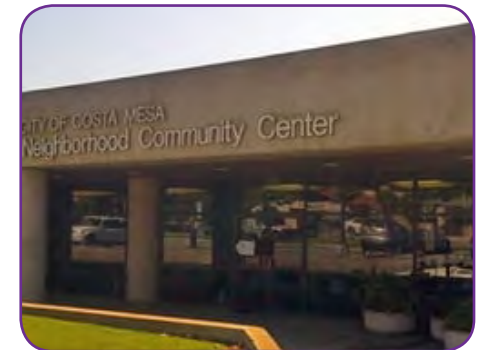
Figure 4-13 Costa Mesa Neighborhood Community Center
