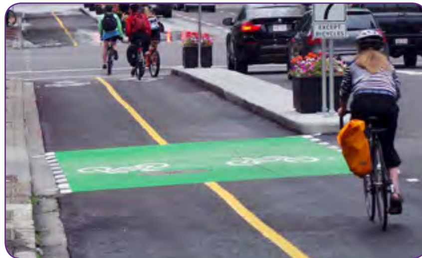
Figure 3-10 Class IV Cycle Tracks
