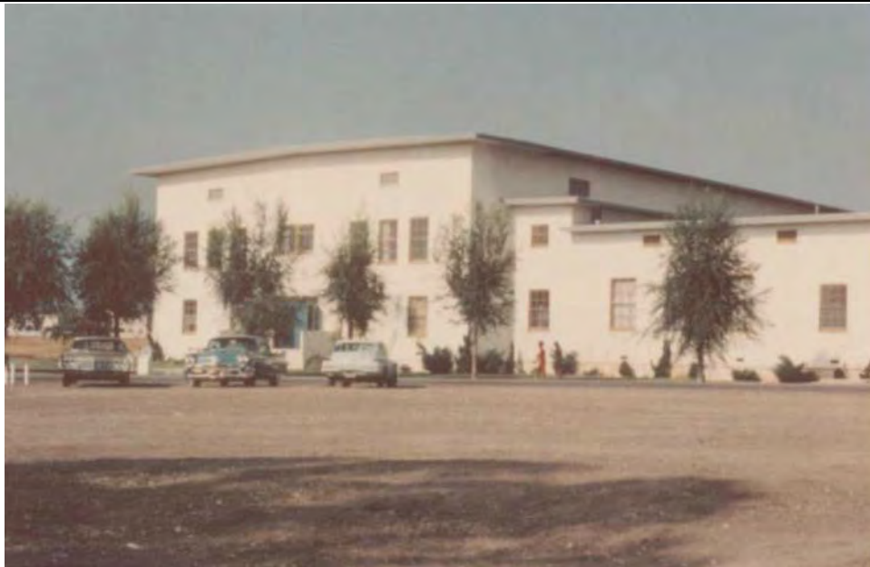
Front (north) elevation of the Gymnasium in 1968. The original fenestration was removed at some point in time. (Source: O. Cope Budge Library Digital Collections)
