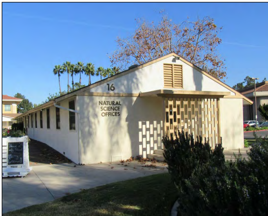
Building 16, one of the original SAAAB barracks buildings, now with stucco siding, modern composite windows and doors, and architectural details added in the 1960s. View looking north.
