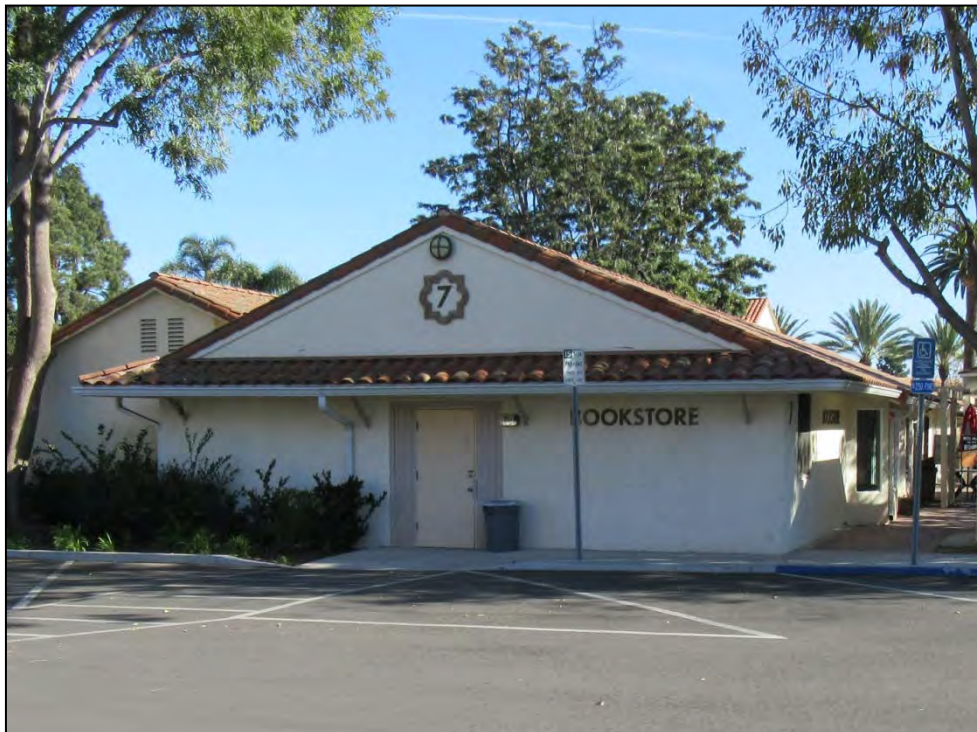
Building 7. View looking east.
