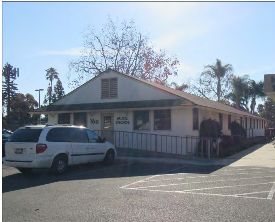
Building 16a. View looking southeast.
