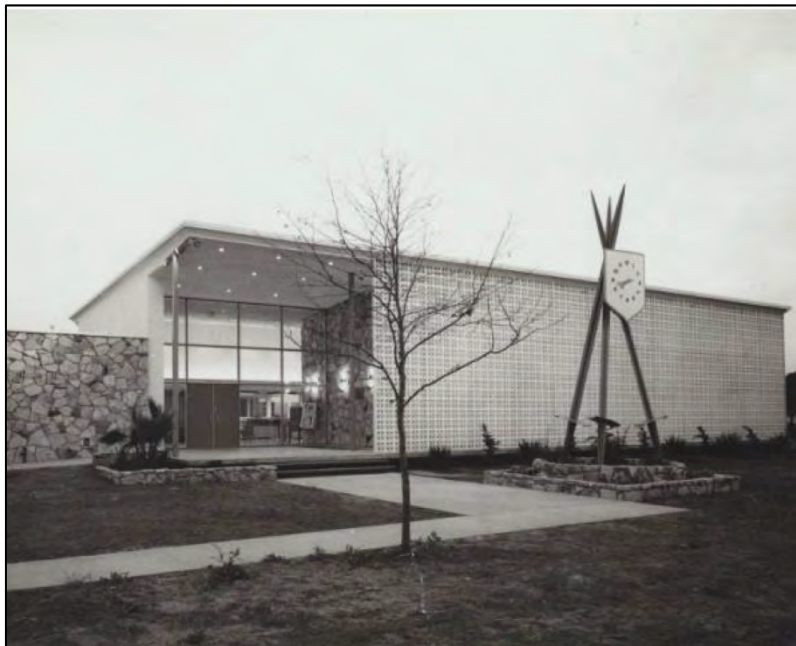
Front (north) elevation of the library when it was completed in 1963. The clock structure was removed in 2008, and the concrete screen across the façade was also removed at some point in time. (Source: O. Cope Budge Library Digital Collections)
