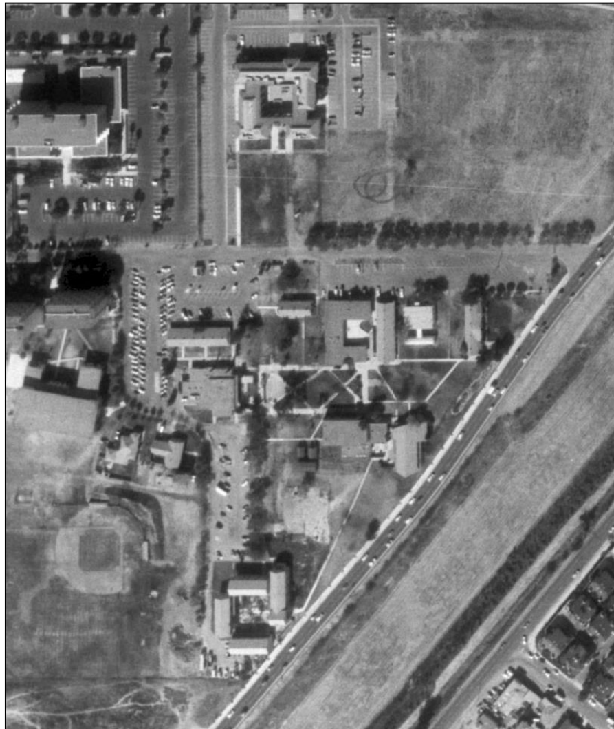
Aerial view (looking north) of the campus of Southern California College in 1980. This was the campus layout prior to the construction of SR 55 and the realignment of Newport Boulevard along the eastern boundary of the campus. The road construction forced the college to demolish and/or move buildings located along Newport Blvd. (Source: NETR Historic Aerials)
