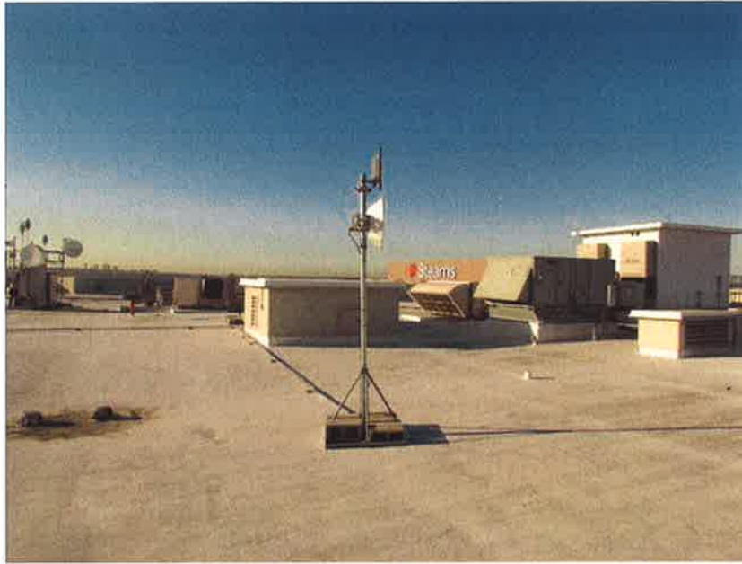
(South View of Existing Equipment)
