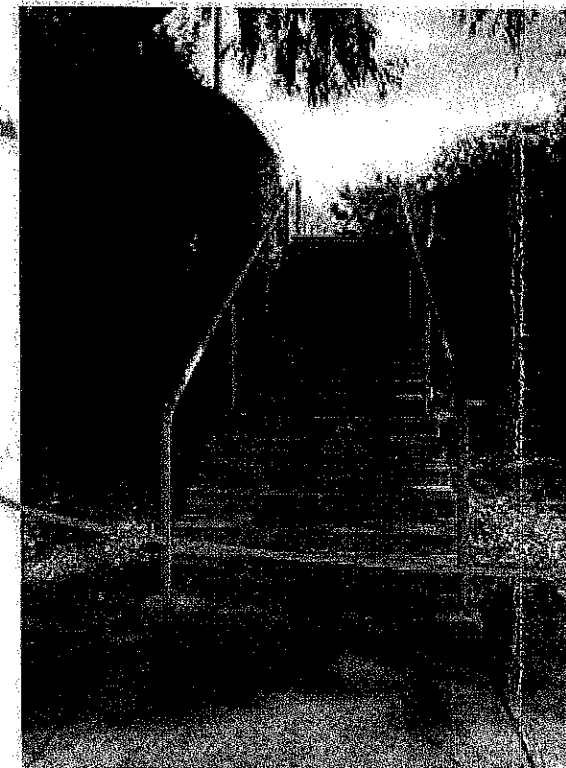
Provide Lighting for Stairway off of Bear St.
