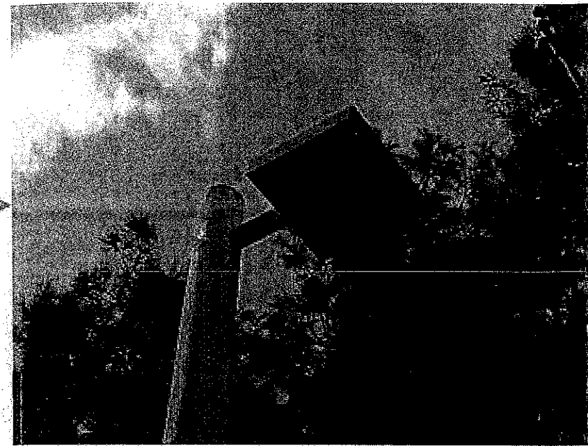
Amphitheatre Light needs Replacing
