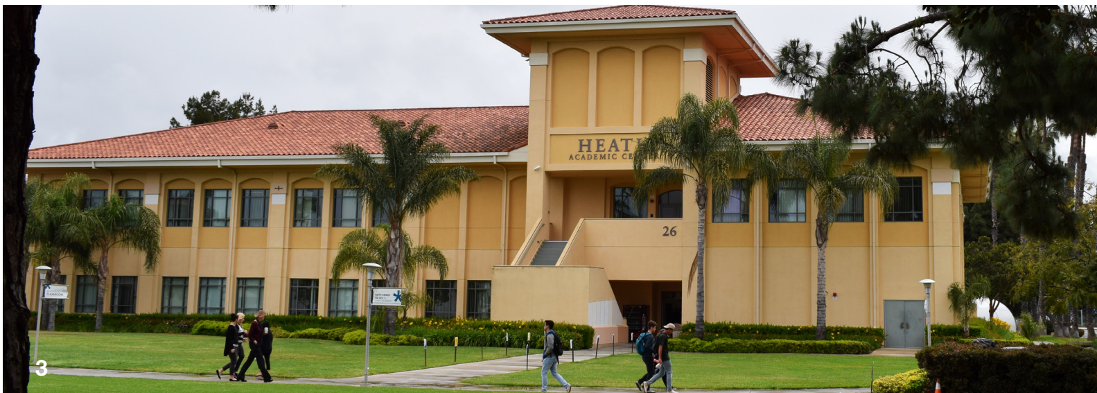
1 THE HIVE Outdoor meeting areas at The Hive a creative office campus. | Steelwave
