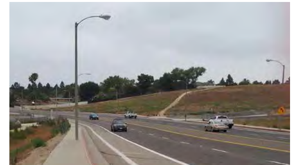
Existing Class II buffered bike lane on Placentia Avenue
