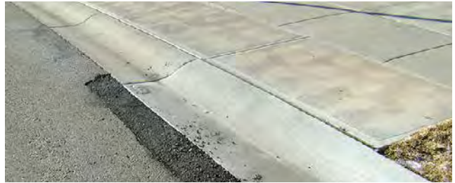
Gutter to Pavement Transition
