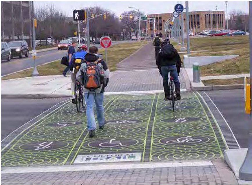
Sample treatment for an Urban Trail crossing at a signalized intersection. Photo source: Richard Layman (Indianapolis Cultural Trail, Indianapolis, IN)
