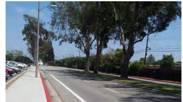
Existing Class II bicycle lane on Merrimac Way
