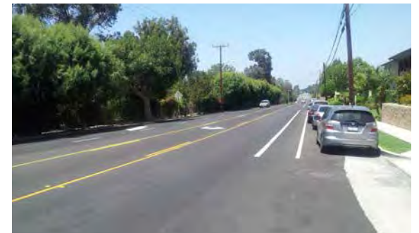
Existing Class II Bicycle lane on Santa Ana Avenue
