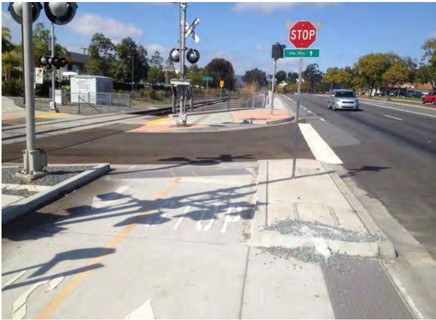
Sample treatment for an Multi-Use Path crossing at a stop-controlled intersection. Photo source: John Holloway (Inland Rail Trail, San Marcos, CA)
