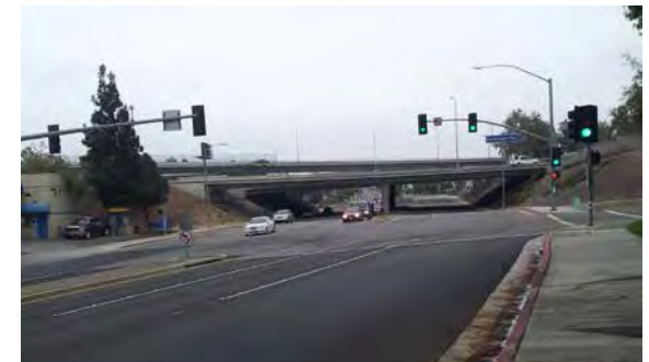
No striped bicycle lanes are provided on Bristol Street
