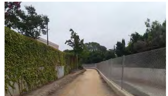
Unpaved multi-purpose trail near Newport Beach Golf Course
