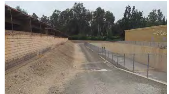
Unpaved maintenance road near Santa Ana Avenue
