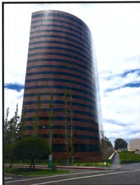
Existing Freestanding Sign and Center Tower
