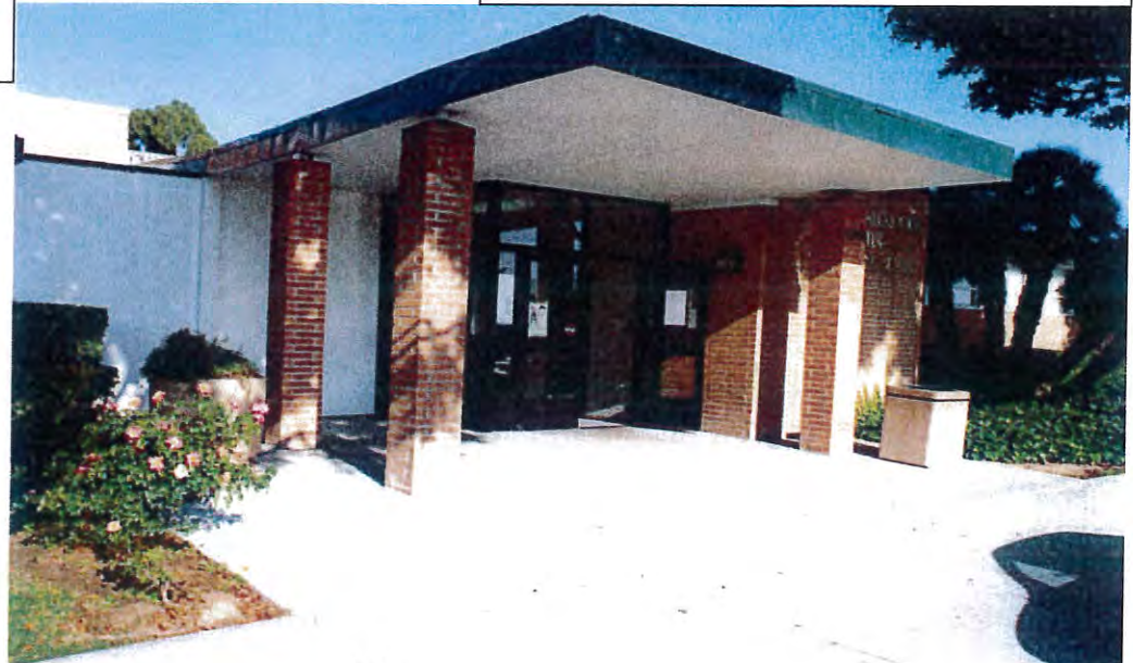
AFTER - New concrete entry slab and removal of steps and rails made the main entry completely accessible.
