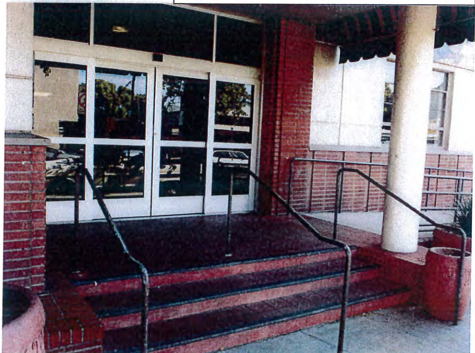
AFTER - New automatic sliding doors and handrails
