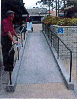
New ADA Compliant ramps & handrails throughout the Civic Center reception counter, restrooms
