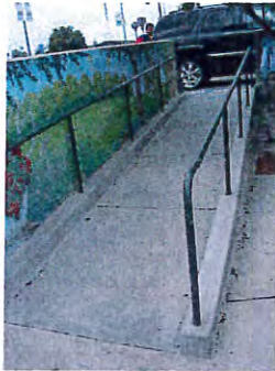
New ADA Compliant ramps & handrails throughout the Civic Center reception counter, restrooms
