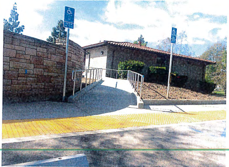
AFTER, new ADA compliant entry ramp
