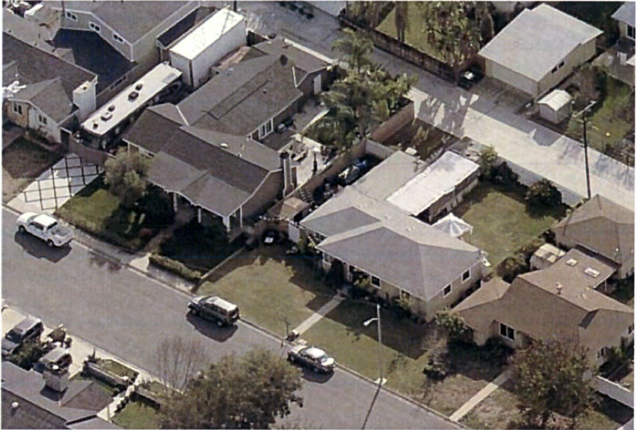
Aerial view of 207 Fairway Place
