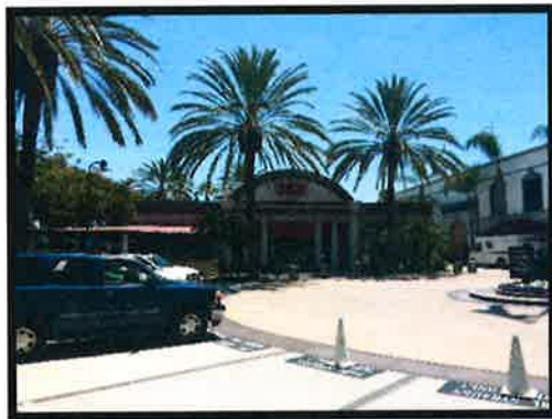
Existing Exterior of Building
