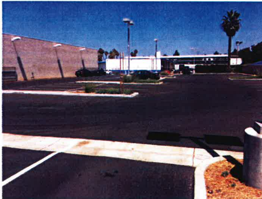
Rear Parking Lot
