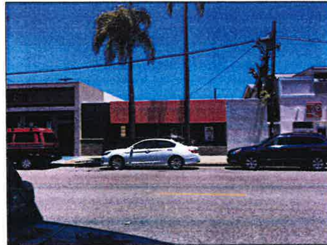
EXISTING FRONT SCALE 1/4" = 1'-0" (C) PHOTO WAS TAKEN PRIOR TO START OF
