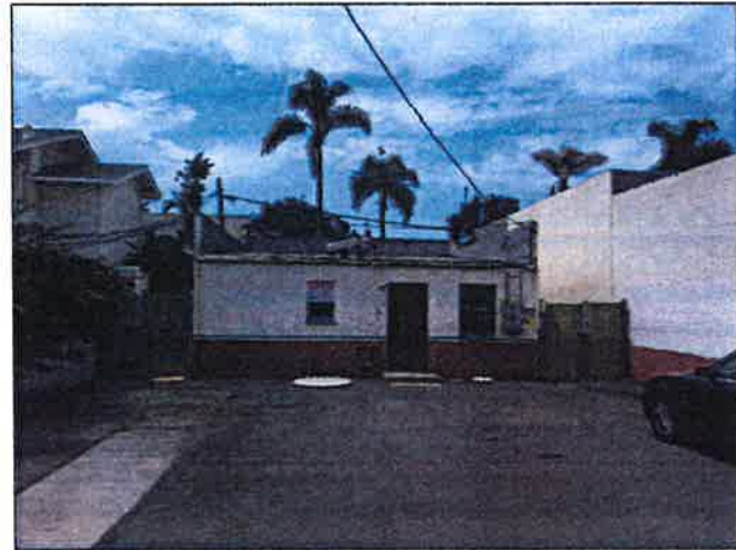
EXISTING REAR SCALE 1/4" = 1'-0" (D) PHOTO WAS TAKEN PRIOR TO START OF CONSTRUCTION ON THE SALON, SALON IS NOW UNDER CONSTRUCTION
