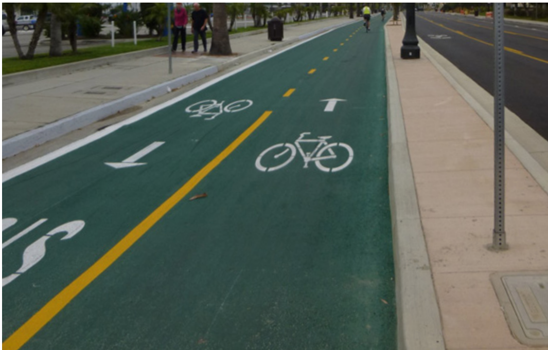
Two-Way Cycle Track (Separated Bikeway) Westwood Blvd, Redondo Beach (Photo: Jim Lyle)
