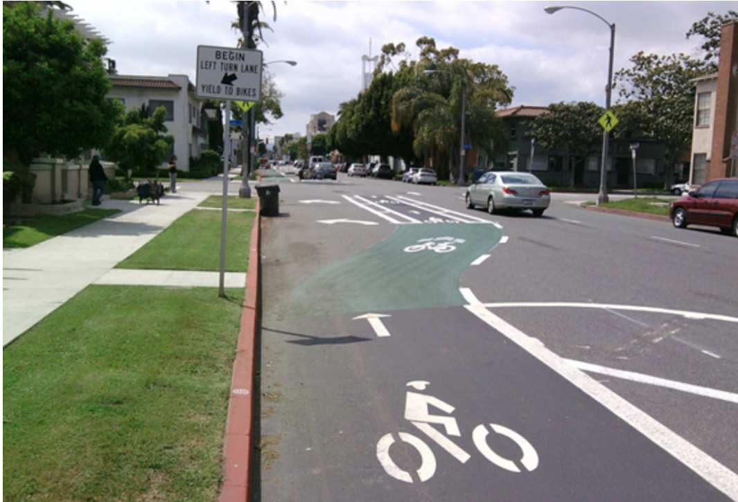
Colored Bicycle Lane in Conflict Area on 3rd St at Lime Ave, Long Beach (Photo: Streetsblog)
