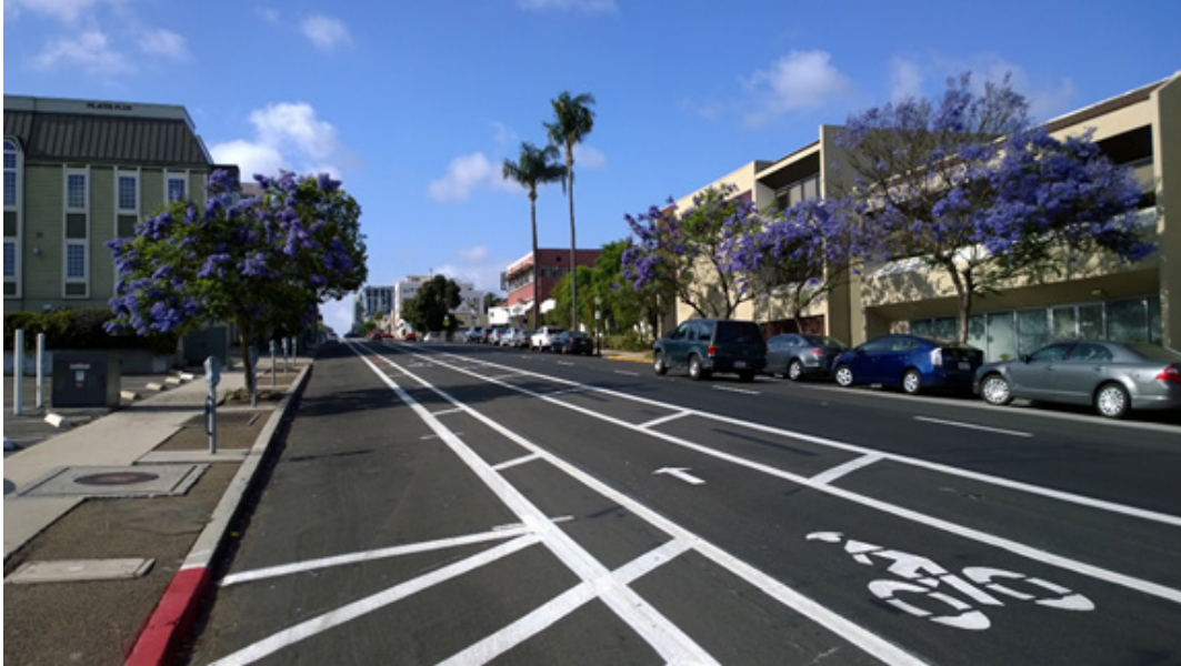
Parking Side and Travel Side Buffered Bike Lane on Fifth Ave, San Diego (Photo: Paul Jamason)
