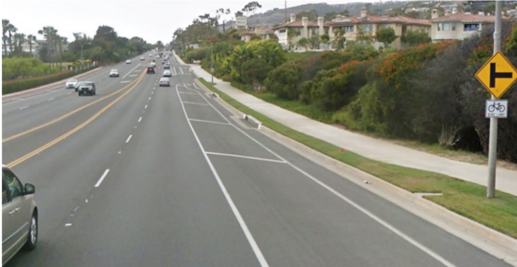
Travel Side Buffered Bike Lane on PCH (SR-1), Dana Point (Photo: Google Street View)
