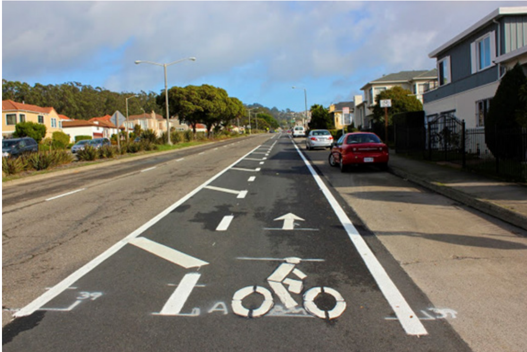
Travel Side Buffered Bike Lane on Sloat Blvd (SR-35), San Francisco (Photo: Mark Dreger)
