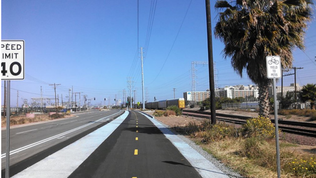
Two-Way Cycle Track (Separated Bikeway) along Harbor Drive, San Diego (Photo: Stephan Vance)
