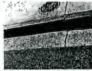
EXISTING CATCH BASIN / EDGE CRACKING AND SETTLEMENT
