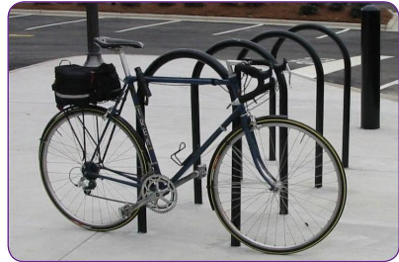
Figure 3-20 Inverted U Bicycle Rack
