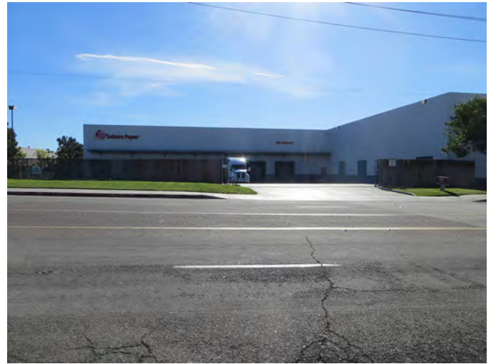
View looking south towards Sunflower Avenue and existing on-site light industrial uses (Sakura Paper Factory).
