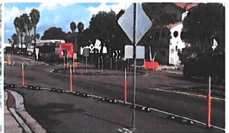
Temporary/quick-build roundabout at 9th & Donax in Imperial Beach (2015)
