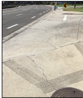
a) South driveway – diagonal ramps
