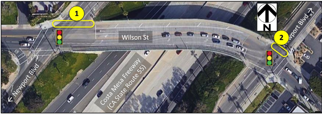
Figure 4-19: Wilson Street at Newport Boulevard – issues and opportunities
