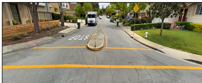
Figure 4-6: Median island on residential street (Canary at Inverness, Sunnyvale CA)
