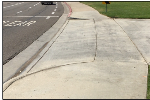
b) North driveway – level bypass (good)
