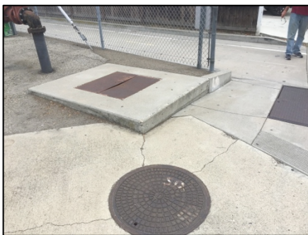
a) View from north
