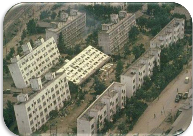
Liquefaction caused by the 1964 Niigita, Japan earthquake caused these apartment blocks to experience severe leaning. Image from the University of Washington.
