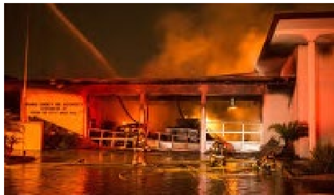
An Orange County Fire Authority station in nearby Buena Park, CA is seen here ablaze in an unexplained 2017 urban fire. Image from Kevin Warn
