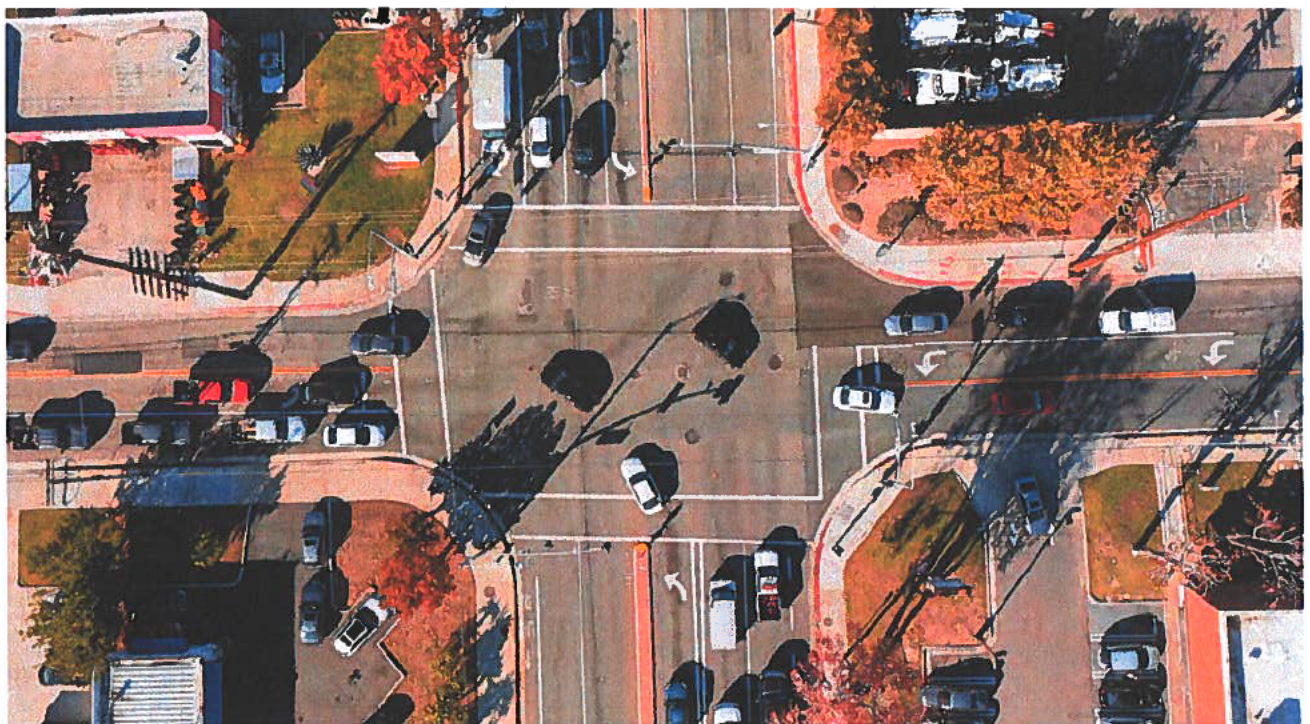
The intersection of Wilson Street and Fairview Road would benefit from updated crosswalk markings and upgraded ADA ramps to improve pedestrian visibility and safety through the intersection.
