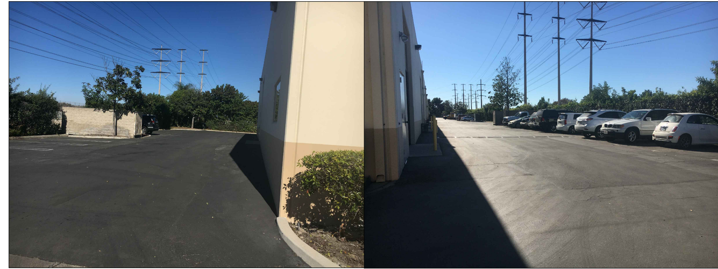
PHOTO #1 - WEST SIDE YARD DRIVE
