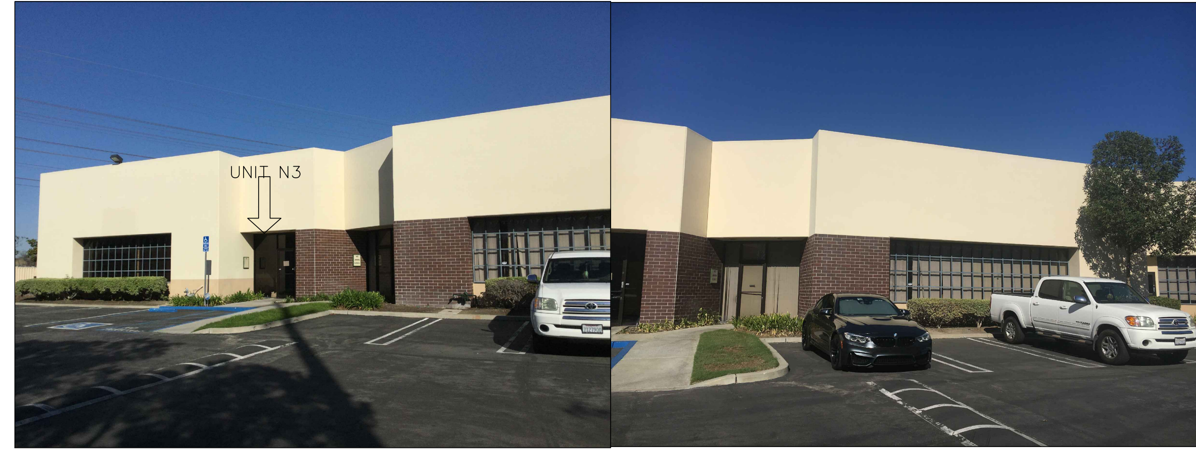
PHOTO #3 - SOUTH ELEVATION ENTRY
