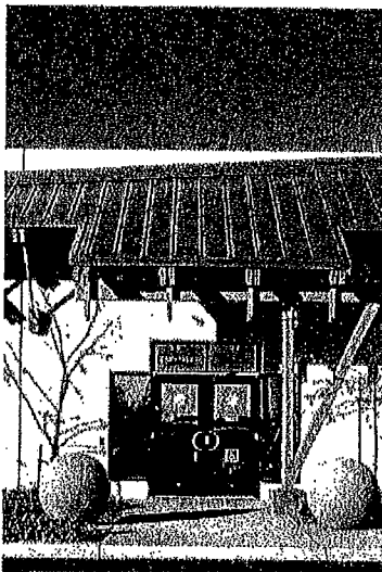
view of building entry
