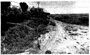
The existing ditch is heavily vegetated and there seems to be no positive drainage pattern. An analysis of the capacity of the existing dirt ditch will be an initial step. The location and alignment of the existing high pressure gas line and overhead power lines will be critical to the preliminary design and alignment of any proposed improvements.
